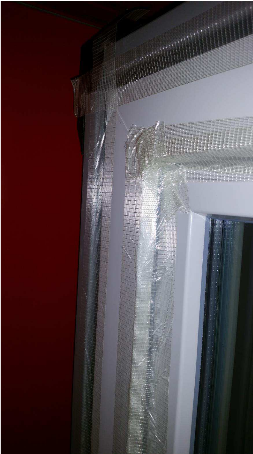
Fig. 2: Sealing of Window and window joints.outside
