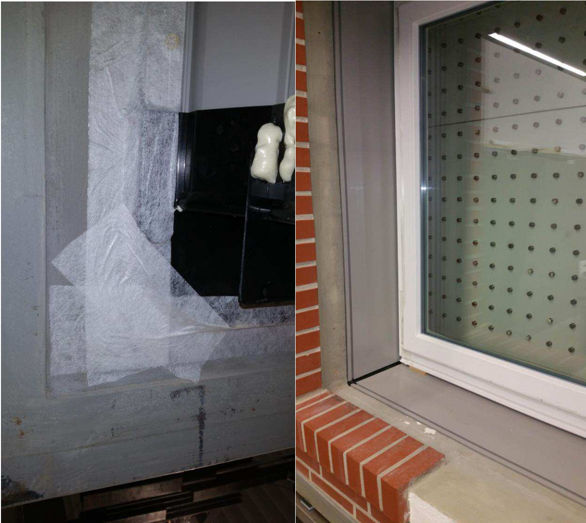
Fig 3: Left: Sealing the OuterCore – Wall joint with Hanno®-Folienband DUO Easy
